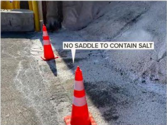
No physical barrier keeping road salt in the Salt Shed. During flood events, water reached the shed & leaches salt
