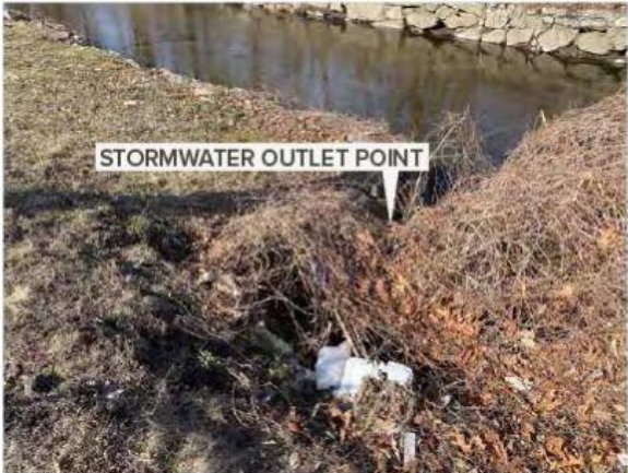
Storm outfall areas are grown over & blocked
