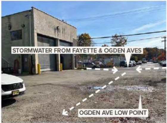
Degraded condition of asphalt show evidence of high stormwater flows
